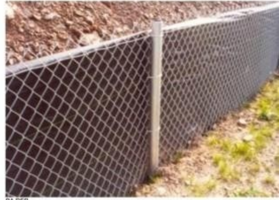
Super Silt Fence Source: PADEP 2012, p.82
