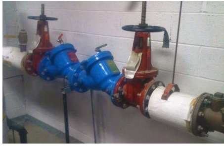
Figure 9 – Example of a Backflow Prevention Assembly
